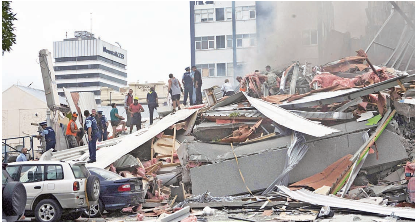
IN A SHAMBLES: Rescue workers search for survivors at the collapsed CTV building that housed the King's Education School in Madras Street in Christchurch, yesterday. - Reuters
