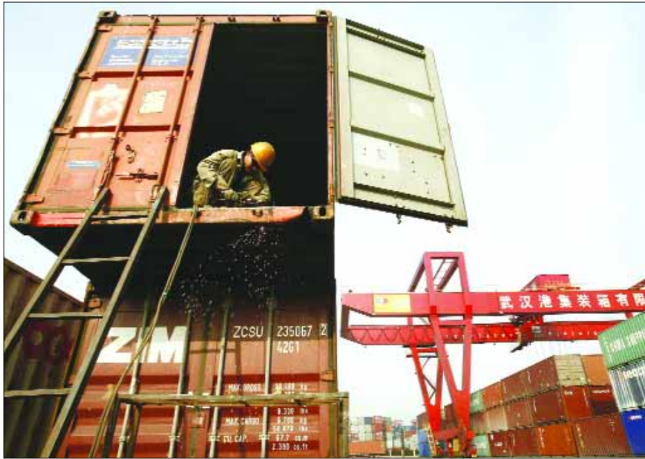
SURPLUS VALUE: A labourer welds the edge of a container at a port in Wuhan, Hubei province, yesterday. China's trade surplus will rise more than 20 per cent this year even though export growth will slow due to weaker demand from the United States, a government researcher said. — Reuters
