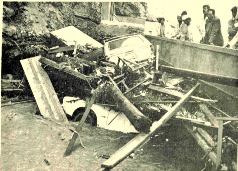
Damages Rain in Muscat
